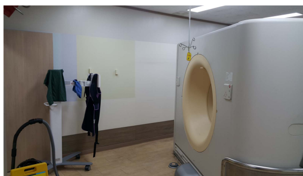
Fig. 4. (Color online) Installation location of the glass dosimeter for user factor analysis for calculating the radiation shielding facility protective wall.
