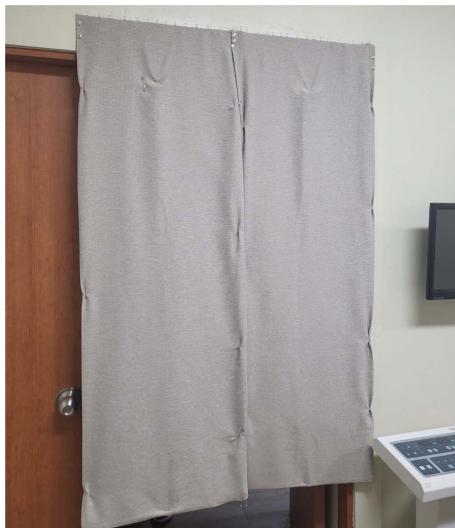
Fig. 4. (Color online) Image of a lead curtain hanging over the door of a diagnostic electromagnetic radiation generator.
