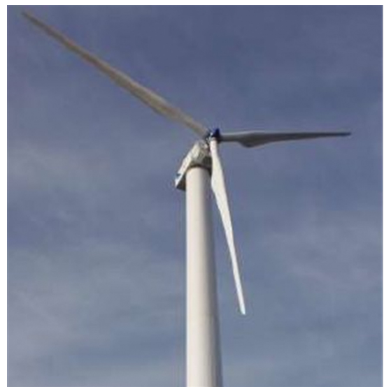
Fig. 3. (Color online) Seoltech, 100kW-Class Wind turbine generator (Direct-Drive 50 rpm, 24.4 m × 11.7 m) [9].
